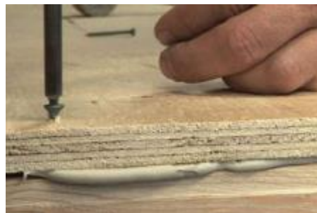
Figure 03 – Securing the Substrate to the Joist System
