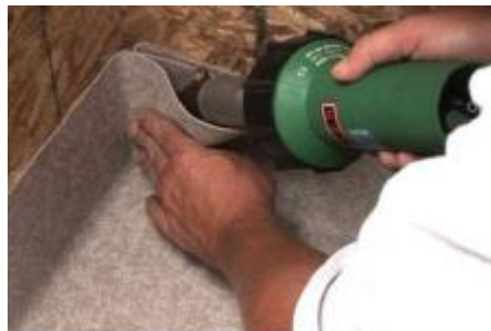
Figure 28 – Sealing the Pigs Ear
