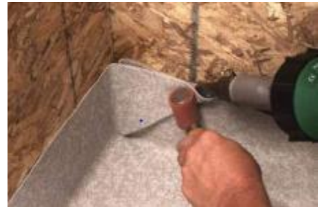
Figure 29 – Thermally heat welding the Pigs Ear to the Wall
