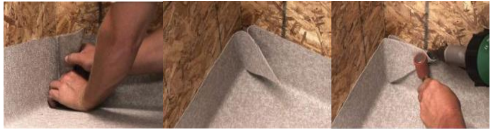
Figure 21 – Fitting an Inside Corner (Pigs Ear Detail)
