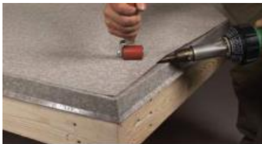
Figure 23 - Thermally heat welding the field membrane onto the Dec-Clad Drip Edge
