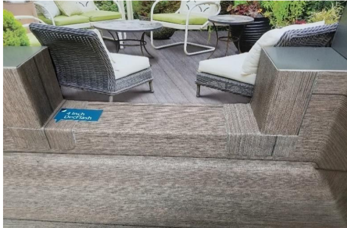
Figure 30 – Typical Threshold Detail using Dec-Flash
