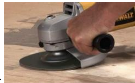
Figure 16 – Sanding the deck surface
