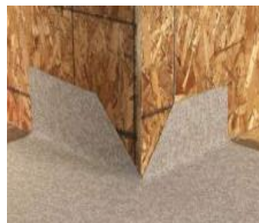
Figure 20 – Fitting an Outside Corner
